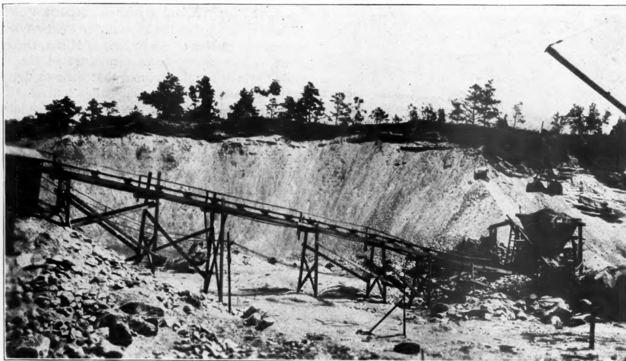
Hopper Loaded by the Bucket at Right and Conveyor to Scalping Screen
